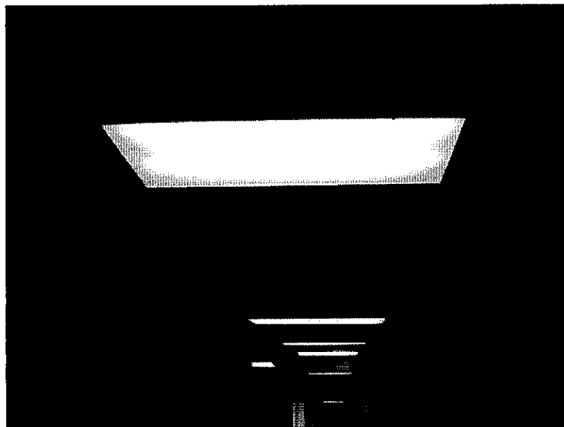
Typical corridor lighting
