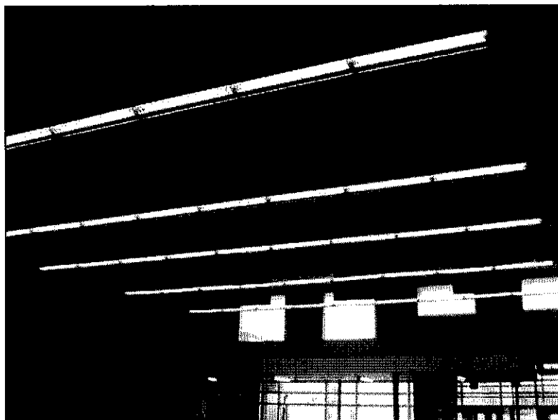
Typical commons area lighting
